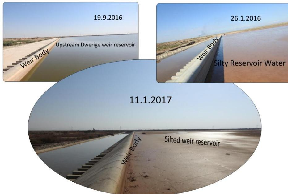
**Fig. 1: Siltation in Dwreige weir during first operating year**
